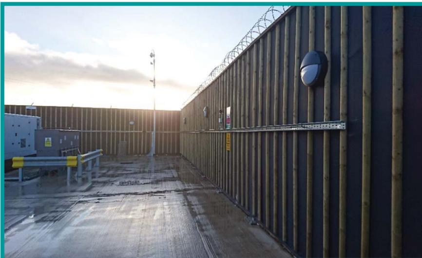
The JCW Absorbent Sound Screen conforms and tested to BS EN 1793. Also tested and complies to BS EN 1794-1 and BS EN 1794-2.
